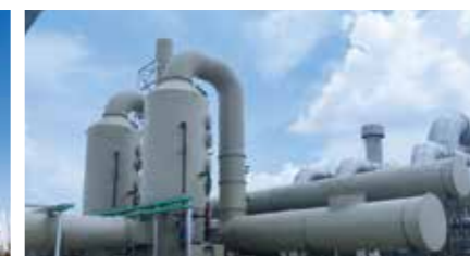
Treatment of acid and alkaline exhaust gases in the semiconductor industry Scrubber
